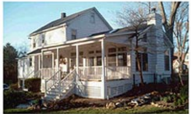
The room is designed to exceed the customers desires and to retain the charm of the original home.
